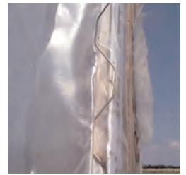
Figure 10. Wiggle (zigzag) wire is used to secure the plastic to the frame.
