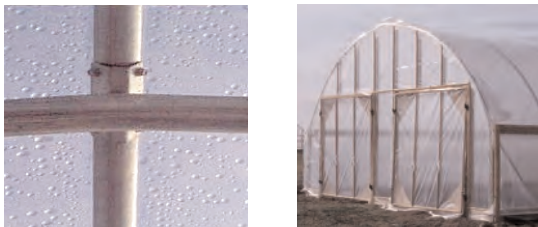
Figure 3. A purlin bracket (left) is used to connect the two bow sections. The center purlin of the Stuppy “Polar Cub” design (right) sits on top of the bows .
