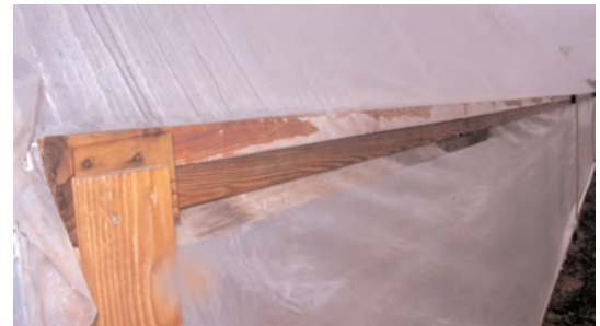
Figure 6. Plastic attached to hip board.
