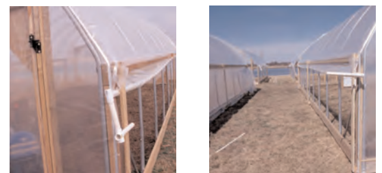
Figure 11. A \frac{3}{4} -inch PVC t-handle (left) rolls the sidewall vents up (open) or down (closed).
