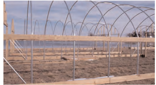
Figure 5. Baseboard and hip board attached to side posts.
