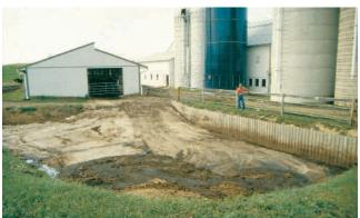
Figure 1. Picket dams provide storage for manure while allowing water to drain away.
