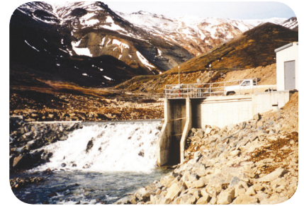
Photo credit: DOE NREL
