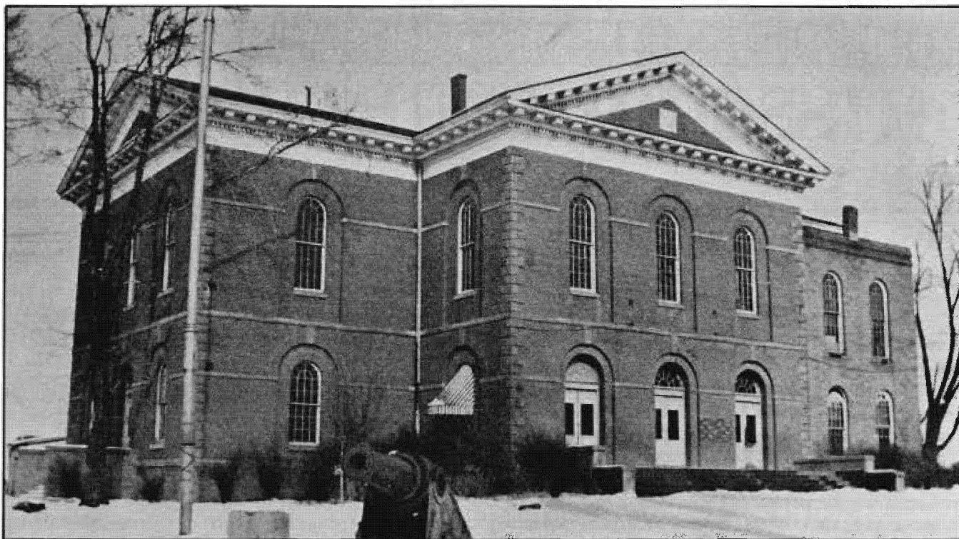
Fig. 2. Platte County Courthouse, 1866-. Architect: Peter McDuff (From: W.P.A., Historical Records Survey)
