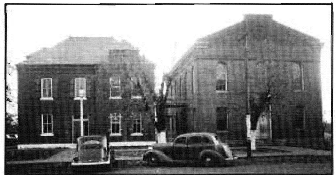
Fig. 2. 1892 addition on left; courthouse on right. (From: Western Historical Manuscript Collection )
