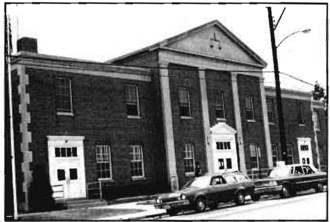
Fig. 4. Jefferson County Courthouse, after 1954 remodeling. Architect: Bruce Barnes and Associates
