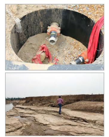
**Figure 20.** The Birds Point Floodway was activated in January, 1937, and May, 2011, by the Army Corps of Engineers. The top photo, taken in 2011, shows a slurry port in an unblown levee section. The bottom photo shows deep soil cuts created by rushing water at O'Bryan's Ridge in the Floodway.
