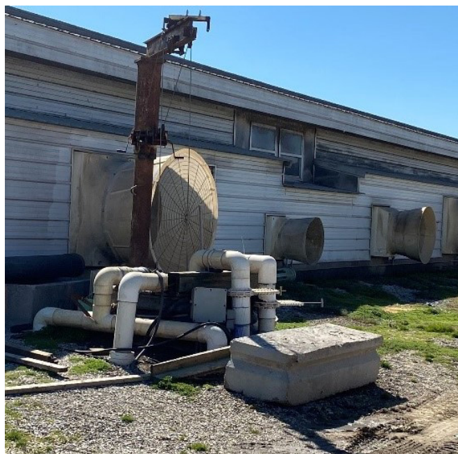
Figure 3. Lift station for pumping recently scraped manure from the finishing barns to the composting facility.
