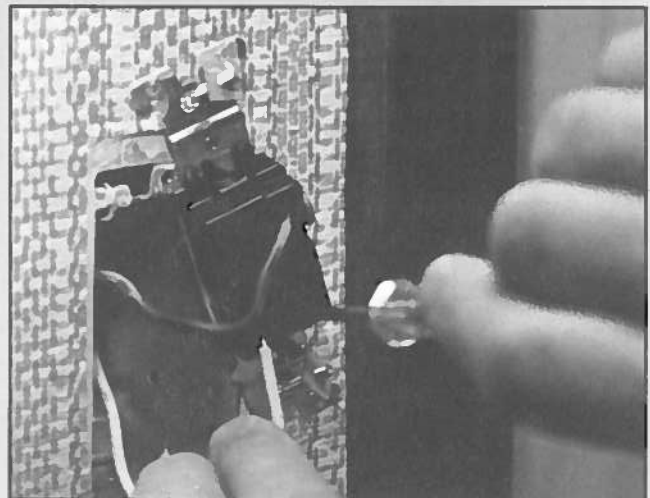
Figure 7. Pushing small screwdriver in slot to release conductor.
