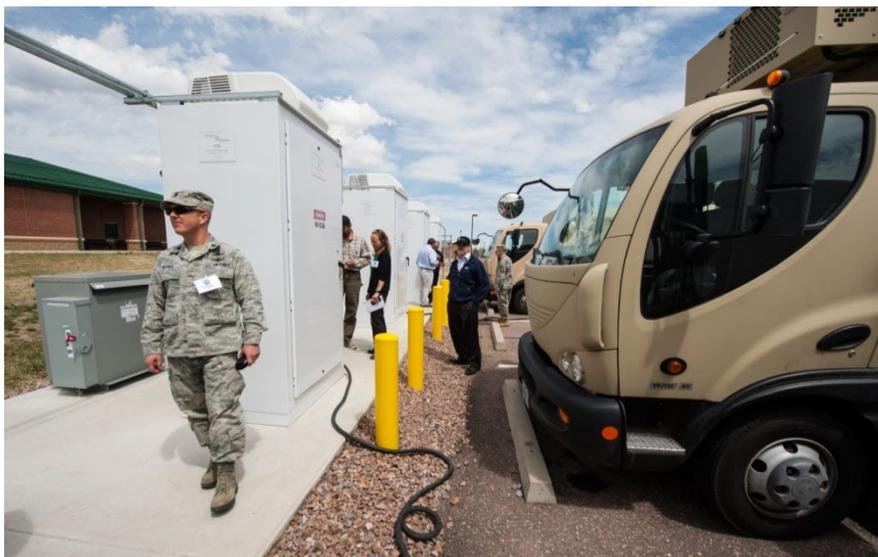
Bi-directional, fast-charging electric vehicle stations are capable of supplying power back to the Ft. Carson Army Base microgrid to help address demand or enhance overall power quality. (Photo by Dennis Schroeder /DOE-NREL)
