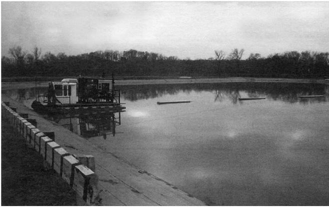
**Figure 2.** The dredge used for removal of biosolids from a lagoon.
