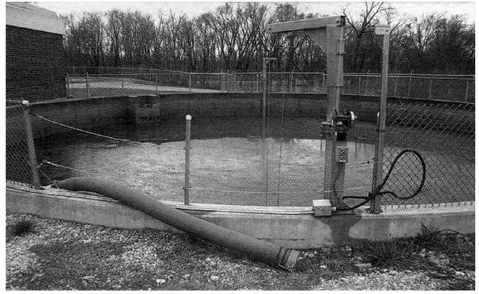
**Figure 4.** Short-term storage tank for biosolids removed from a lagoon.
