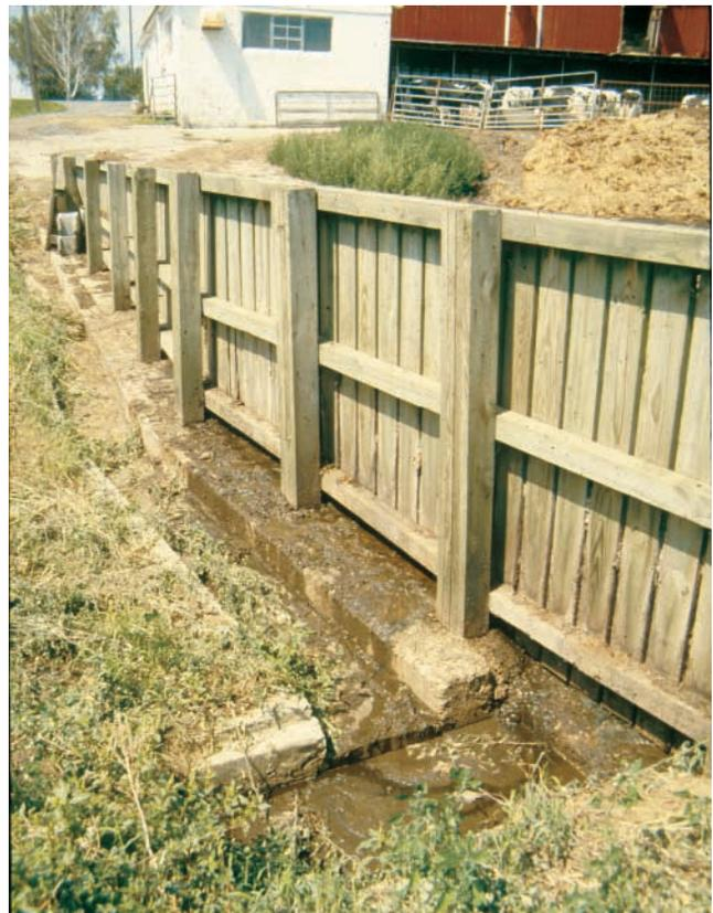
Figure 2. A concrete trough collects runoff that drains through this picket dam.
