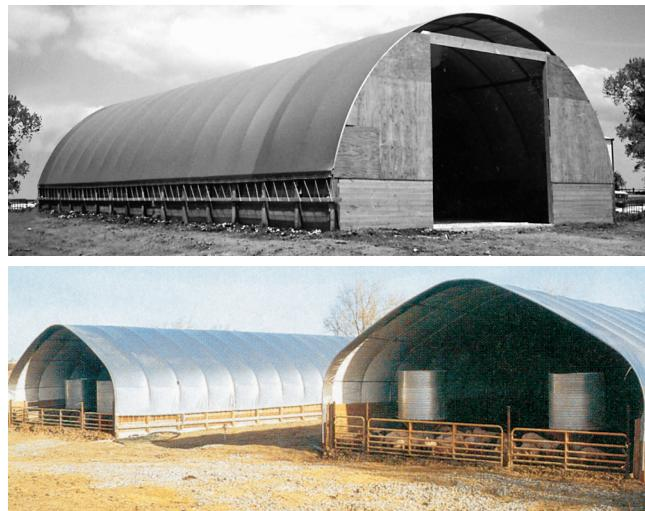
**Figures 1 and 2.** Hoop structures are lower-cost facilities that require bedding and handling of manure as a solid.
