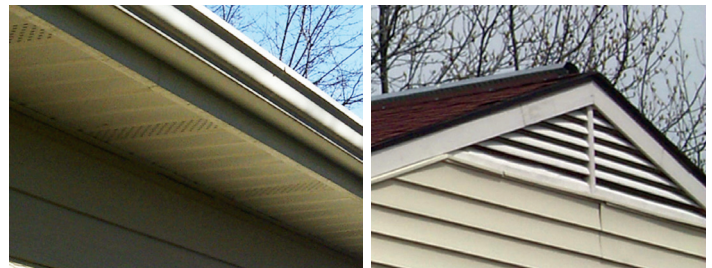
A combination of eave, left, and ridge vents creates a natural convection current, keeping your attic cool and moisture-free.
