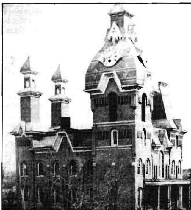
Fig. 3. Randolph County Courthouse, after 1877 remodeling. Architect of remodeling: C.B. Clarke (From: Jason Wright collection)
