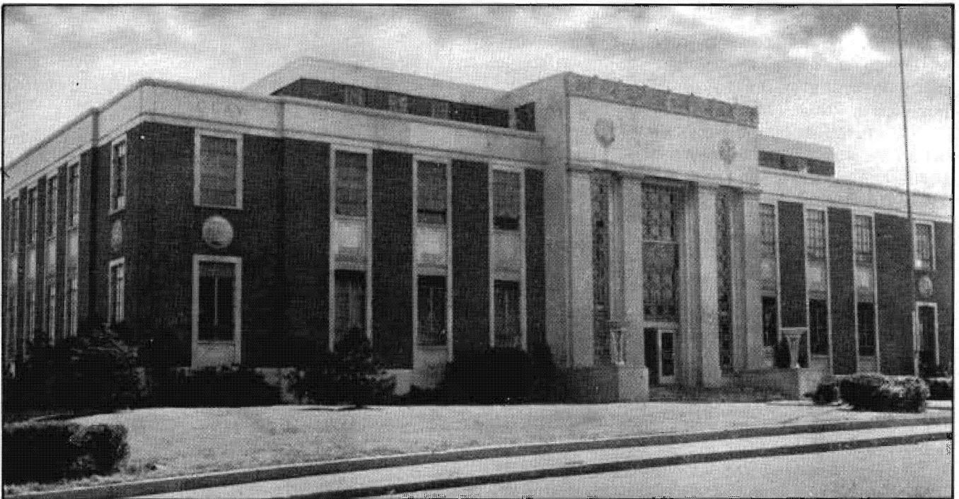
Fig. 3. Callaway County Courthouse, 1938-. Architects: E.C. Henderson, Jr. and Paul Elsner, Fulton: Clark Merrick, Boston. (From: postcard, Trenton Boyd collection)
