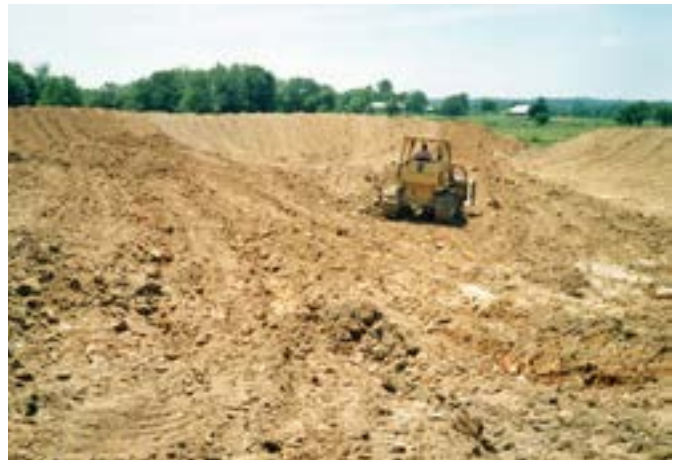
Figure 2. Take special care during the design and construction phases to ensure that the amount of watershed matches the desired pond size.
