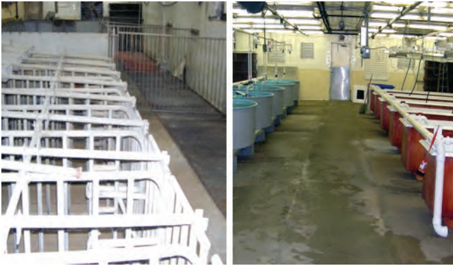
Figure 11. Retrofitting an existing building such as a swine barn (a) for aquaculture production (b) can lead to a profitable enterprise.
