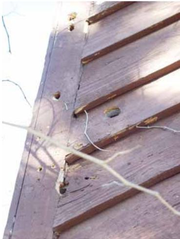
**Figure 1.** Woodpeckers can cause extensive damage to wood siding.
