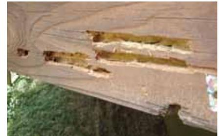
**Figure 3. Woodpeckers may damage wood siding in search of foods such as carpenter bee larvae.**
