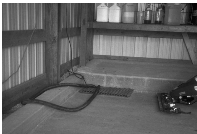
Figure 5. Use nonporous material for storage area flooring.
