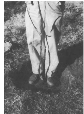
Figure 4. Tamp the soil with your foot as the hole is filled.
