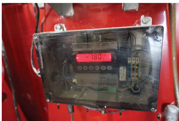
Weigh-Scale display. This scale shows a negative weight which accounts for the weight of the chemical tote.
