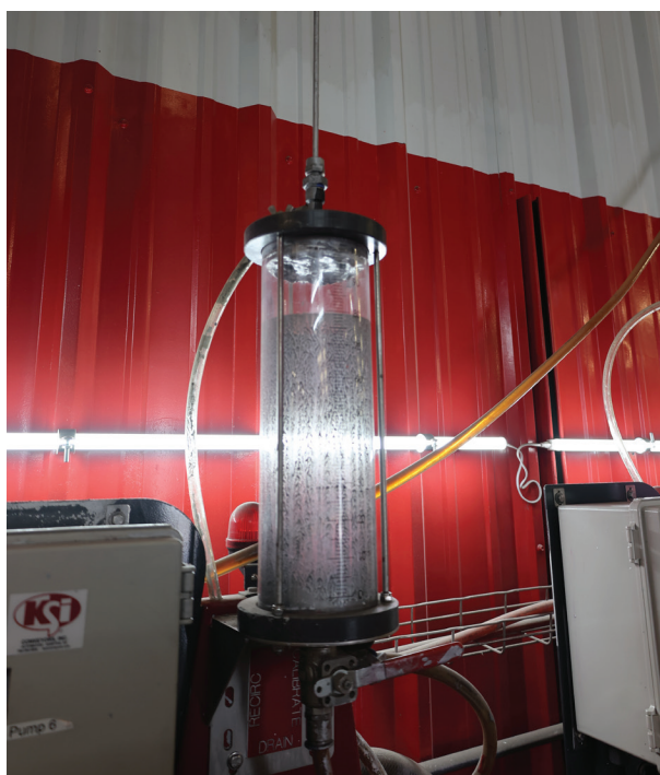
Calibration container. Each station has a calibration container the pump runs into for calibration purposes.
