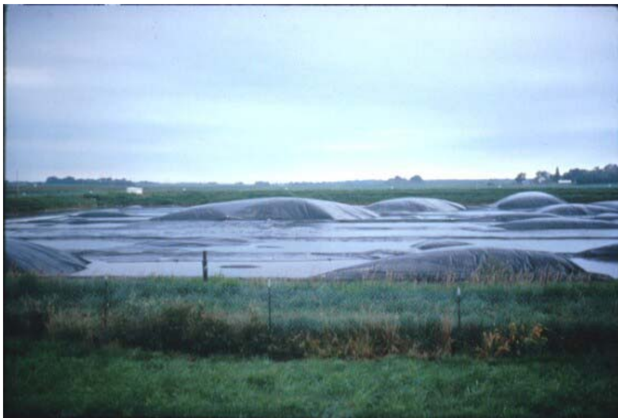
Figure 5-1. Picture of an impermeable cover showing trapped gas “bubbling” the cover and pools of storm water not pumped from surface.
