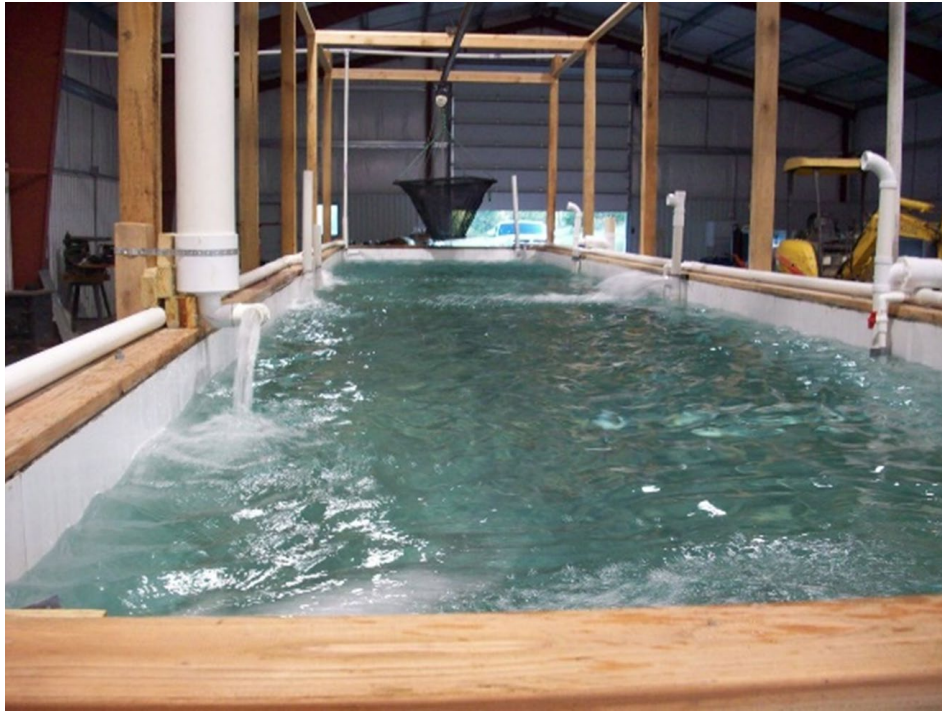
Prefabricated, Concrete-filled PVC Wall-panels
