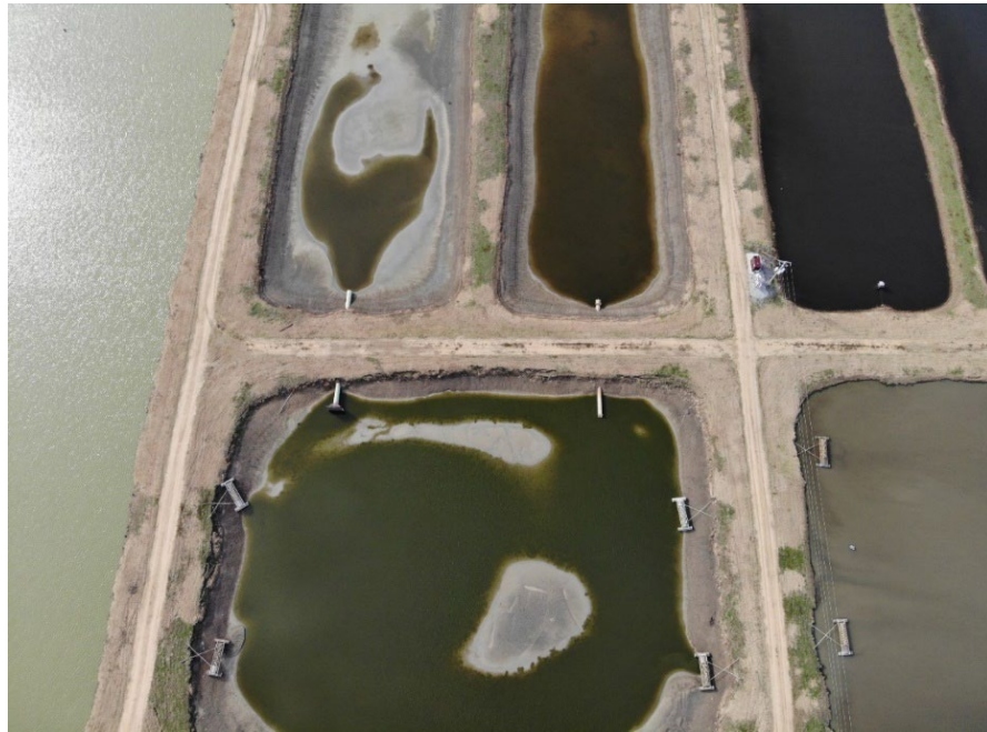
Seven-Acre Split-Pond with Levee in Five-Acre Waste Treatment Zone using Culvert Pumps Delivering 8,000 gpm (11.8 hrs cycle time, \sim 0.0 - 0.048 fps)
