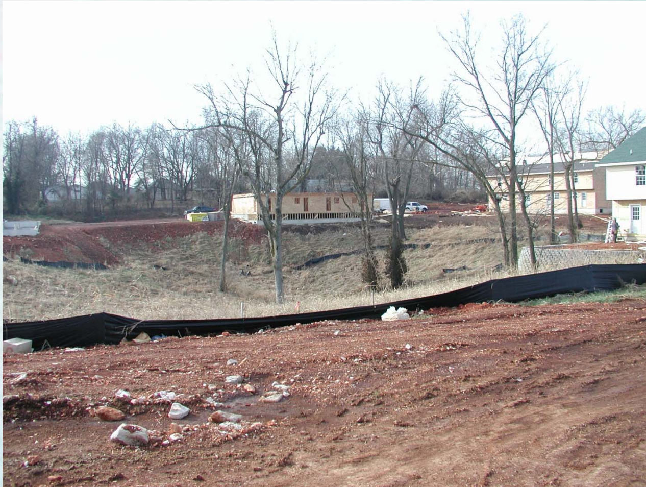
Sinkhole in residential development on SE corner of Kansas Expressway and Walnut Lawn, Springfield, MO
