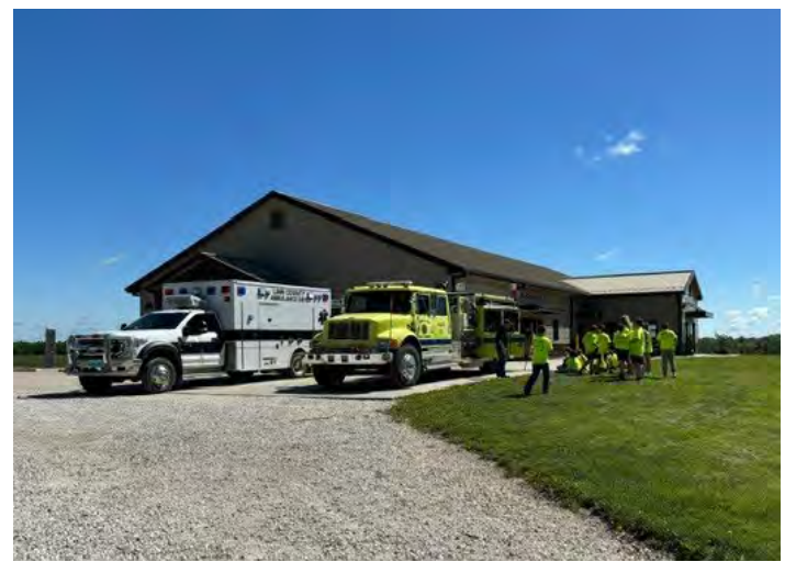
Emergency Vehicle Station
