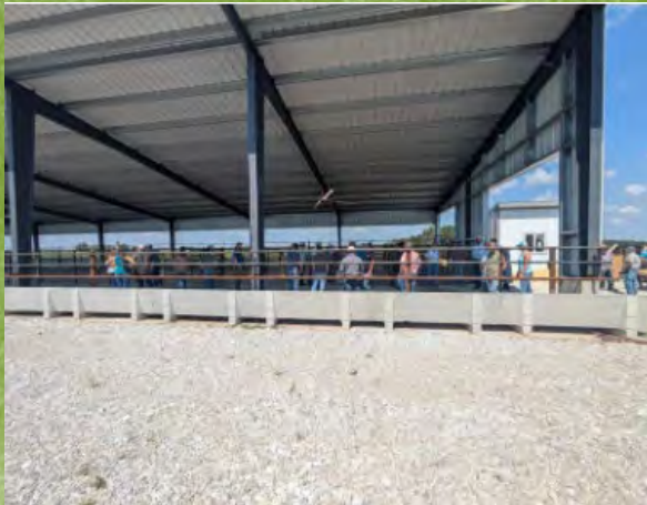
Feedlot Tour of new construction feeding barn in Adair County
