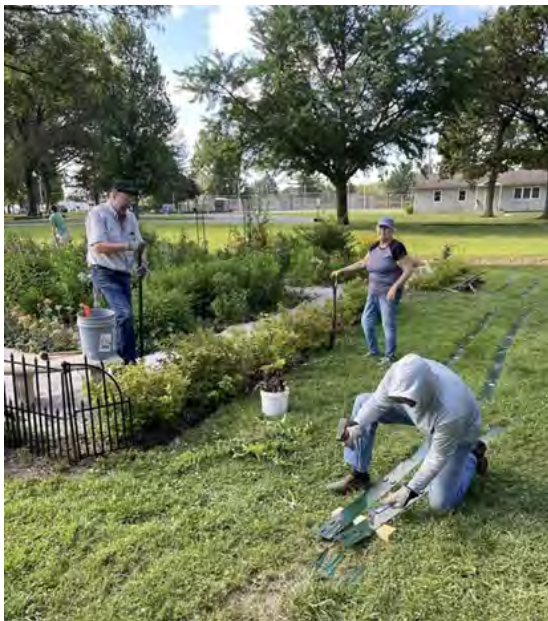
Master Gardeners installing landscape edging around the demonstration Garden at the Lamar City Park.
