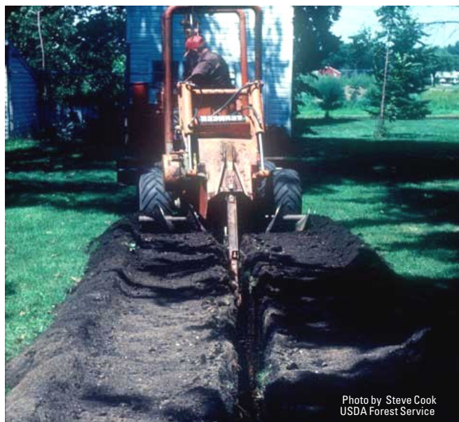
Figure 15. A trenching machine can be used to break root grafts between adjacent oaks of the same species.
