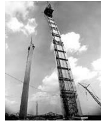
The workmen' elevator car would rise up the creeper derrick track
