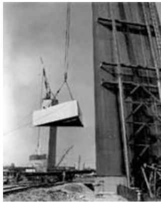
Creeper derricks mounted on tracks lifted most sections
