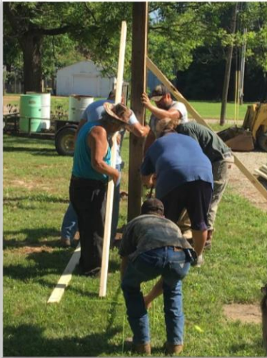
Rombauer Rascals volunteers working on the new pavilion
