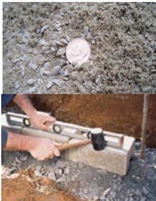
Laying the first row of blocks is the hardest part about installing a retaining wall. It can take up to one third of the time required to complete the entire job.
