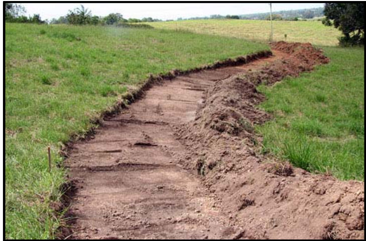
Swale & Berm after Construction (not mulched)
