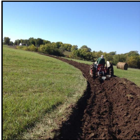
Contour Berm/Swale Construction
