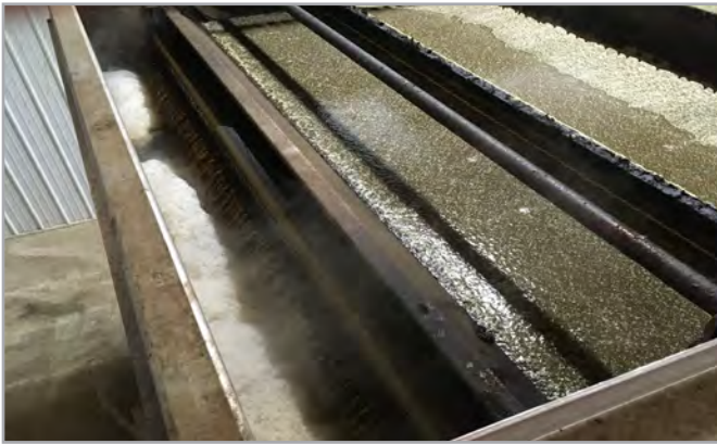
Figure 27. DAF effluent discharge to lagoon.
