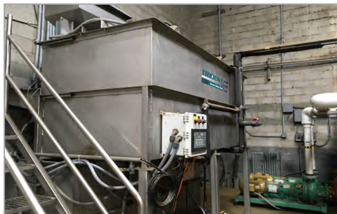
Figure 23. Flocculation tank.
