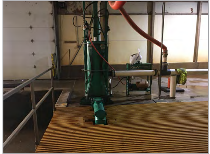
Figure 3. Piston pump.
