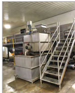
Figure 10. Flocculation and EQ tank with DAF.
