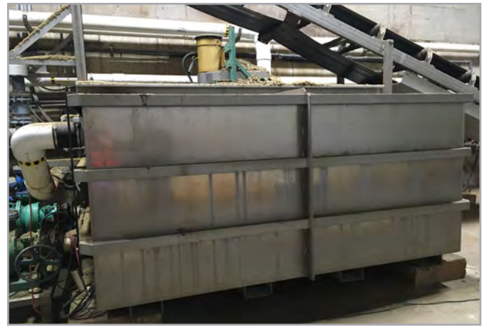
Figure 24. Equalization tank.
