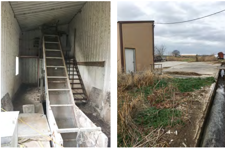
Figure 9. Abandoned manure screen (left) and concrete pad for storing separated solids (right).
