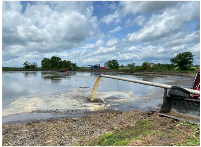
Figure 5. A dilution pump was used to pump water from the nearby lake (left) to the dairy lagoon (right) with agitation boat and lagoon agitation working in the background.
