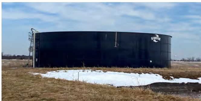
Figure 2. Aboveground slurry tank that was installed at this farm.
