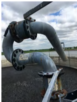
Figure 5. Agitator nozzle located above the slurry tank for breaking up the crust and aid agitation.
